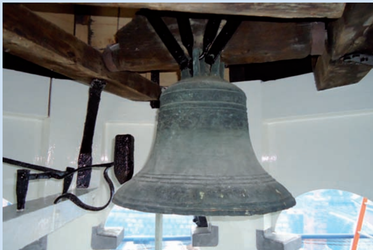
Reset bell (originally from St Leonards Church Corve Street, Ludlow) and hammer, which before it can be rung will have to spring loaded to protect the bell.
