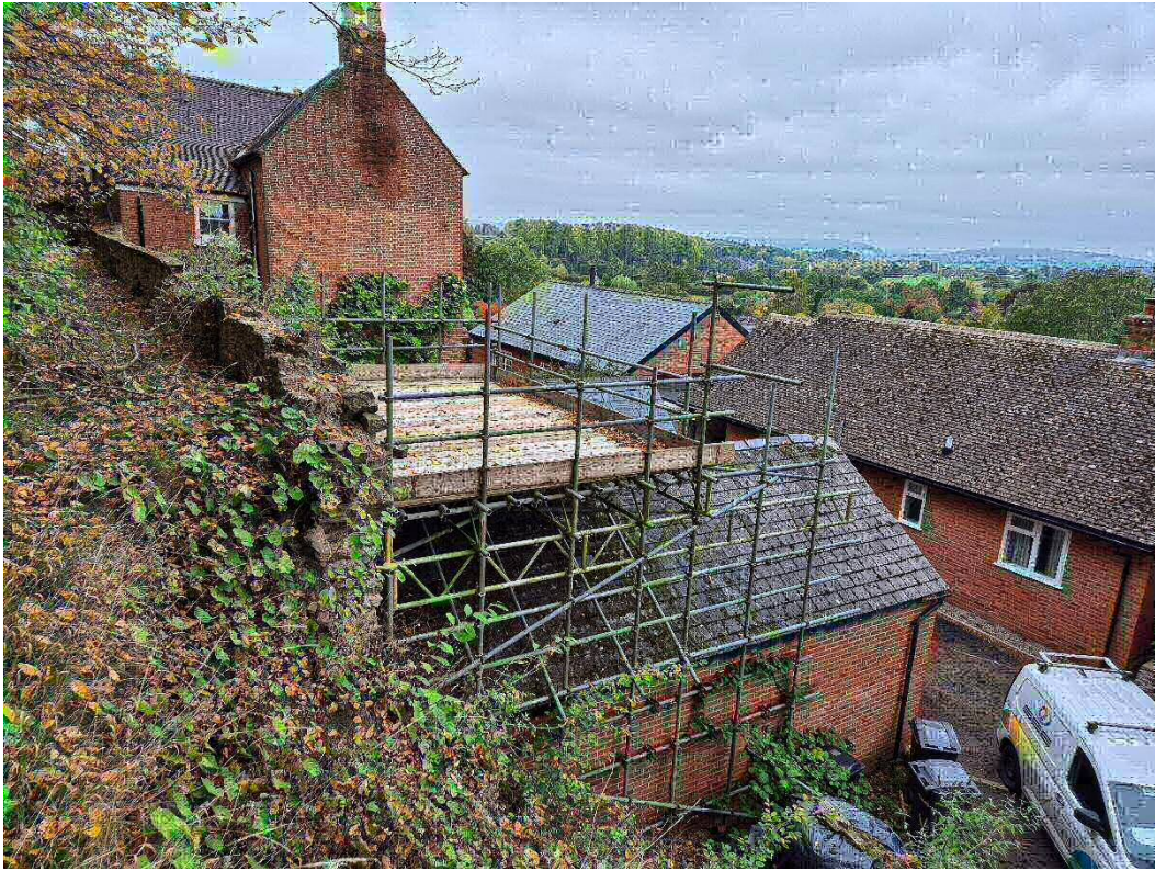
Photograph 1 – Location of scaffolding
