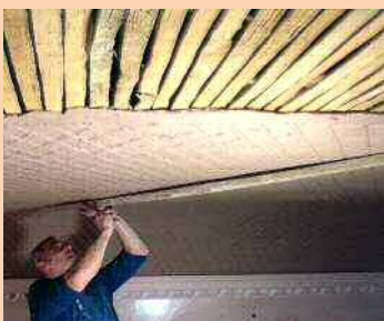
Above - Lime Plastering the ceiling
