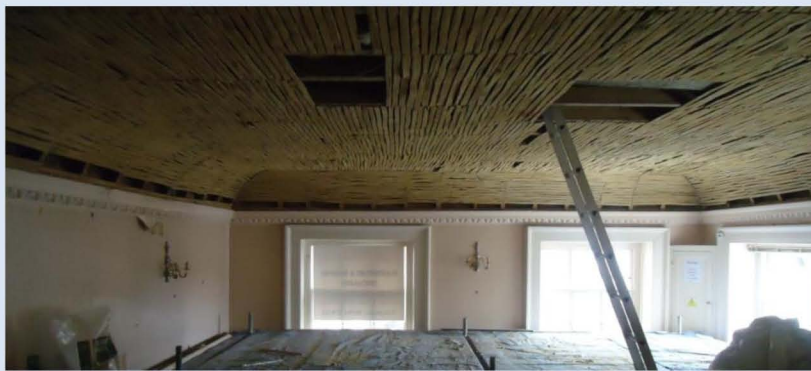
View of Ceiling repair work already began
