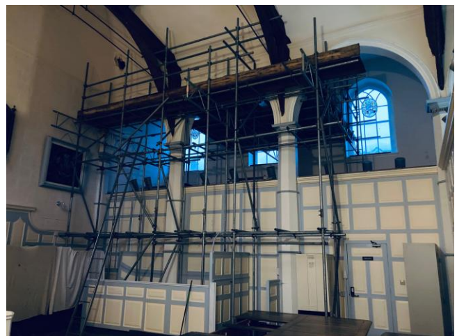
Internal Scaffold at the Guildhall December 2022
