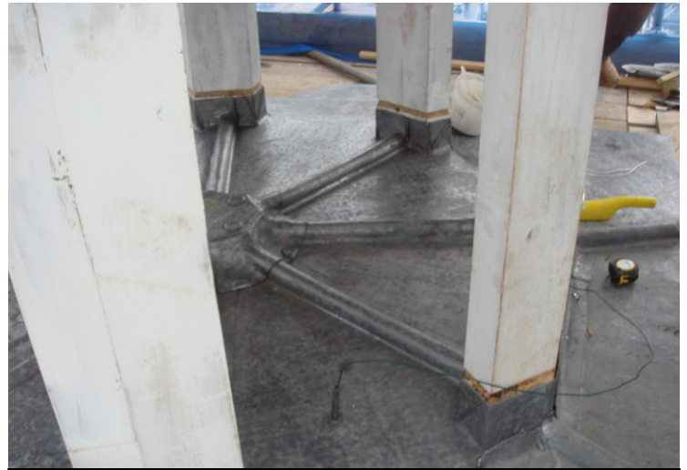
High quality new cupola leadwork
