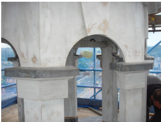
New Cupola render and leadwork
